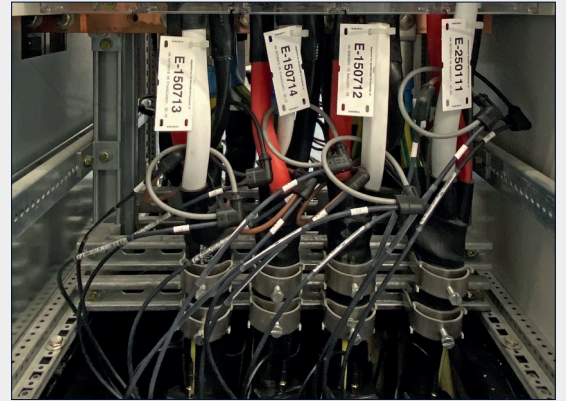
Field installation of Current Link modules
